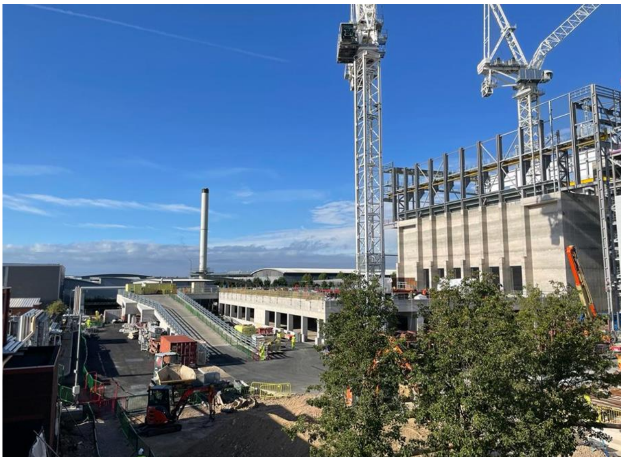
Plate 4.3 – Exit Ramp Concrete Works, Consented Development Construction Works (August 2022)
